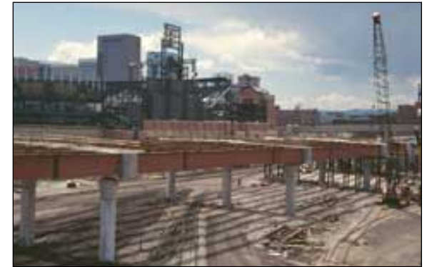
New highway construction near Coors Field
