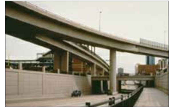
20th Street Viaduct adjacent to Coors Field
