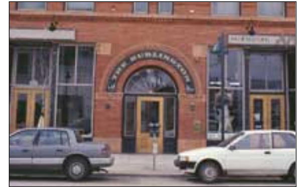
Storefronts in renovated Burlington Hotel building at 22nd and Larimer Streets
