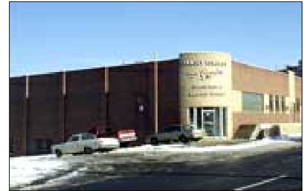
The Pawley Building, at 26th and Walnut Streets, was built in 1948
