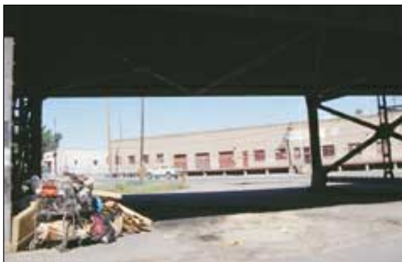
A homeless refuge under the old Broadway Viaduct near Blake Street
