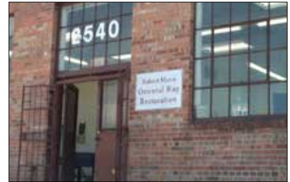
Warehouse reuse at 2540 Walnut Street
