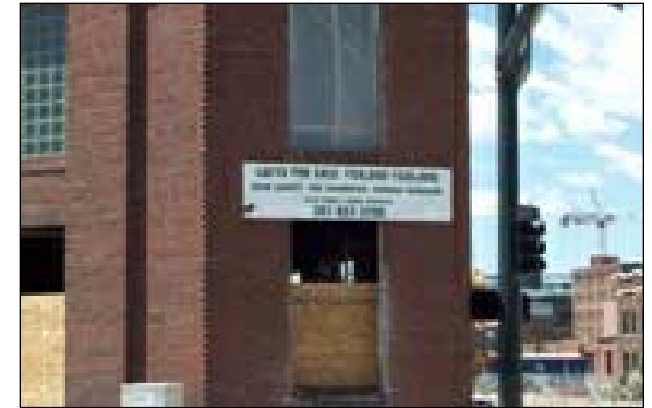
Reuse of industrial buildings to create premium housing along Broadway at Walnut
