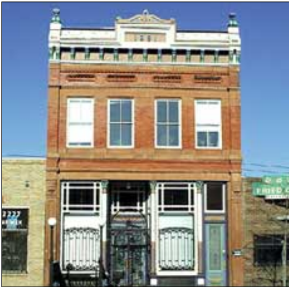
Renovated building on Larimer Street
