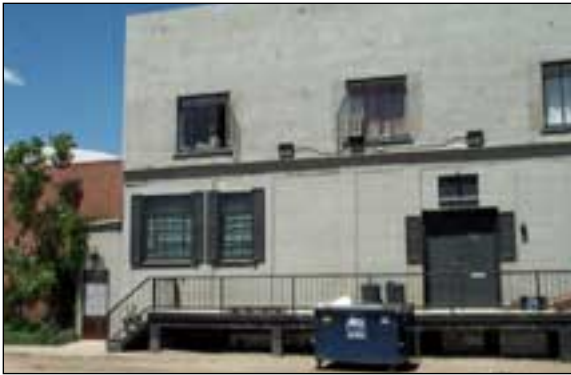
Industrial and residential uses co-exist in Upper Larimer
