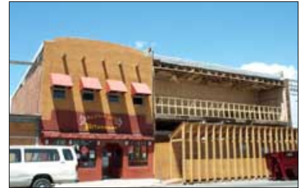
Renovation under way on Larimer Street
