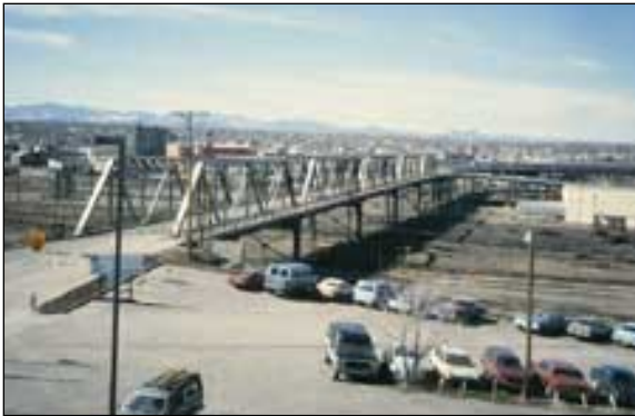
The elevated Broadway/Brighton Viaduct before it was demolished and reconstructed
