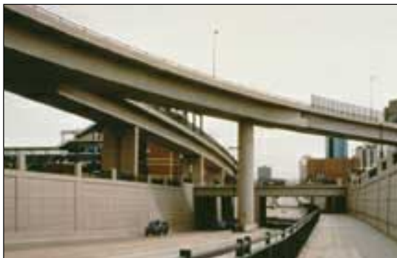
20th Street Viaduct adjacent to Coors Field
